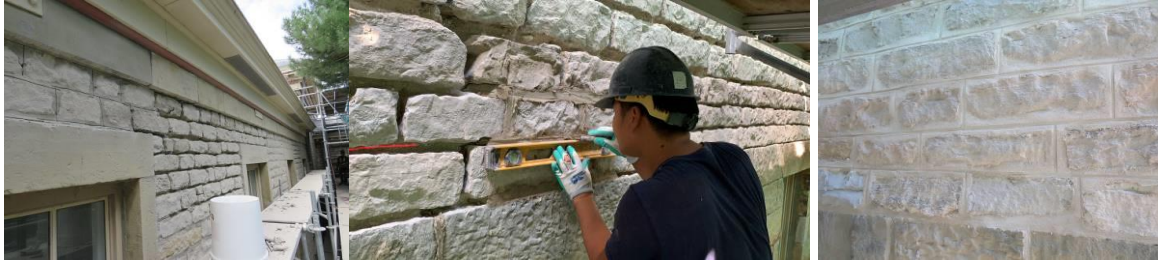
Removal of inappropriate cement mortar for repointing work
