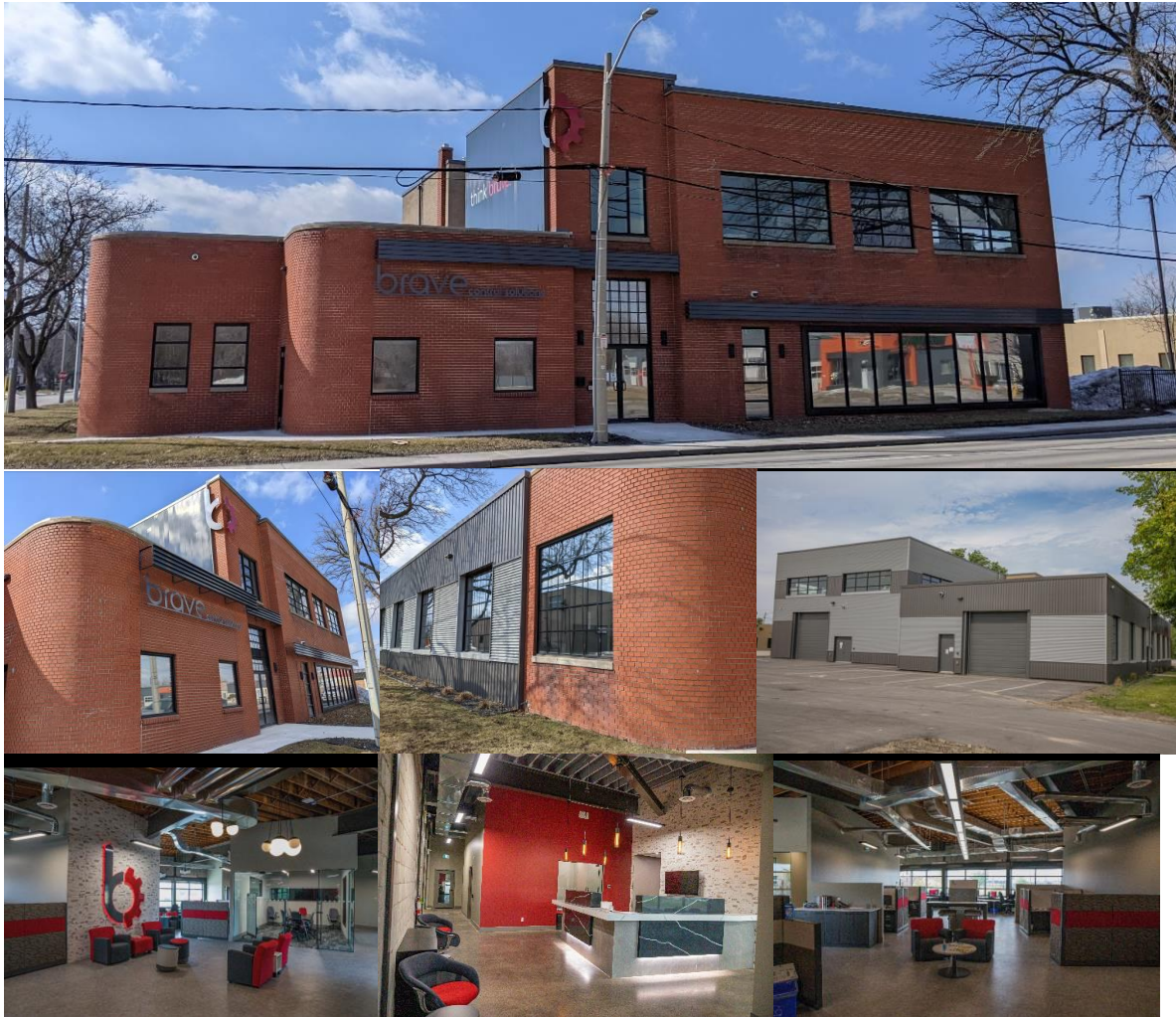
Rehabilitated appearance of the property. (Source: Lester Group)
